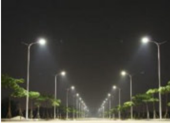
Street lighting upgrades
