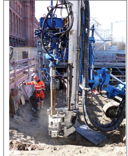
Vibration/rotation drilling head mounted on drilling rig
