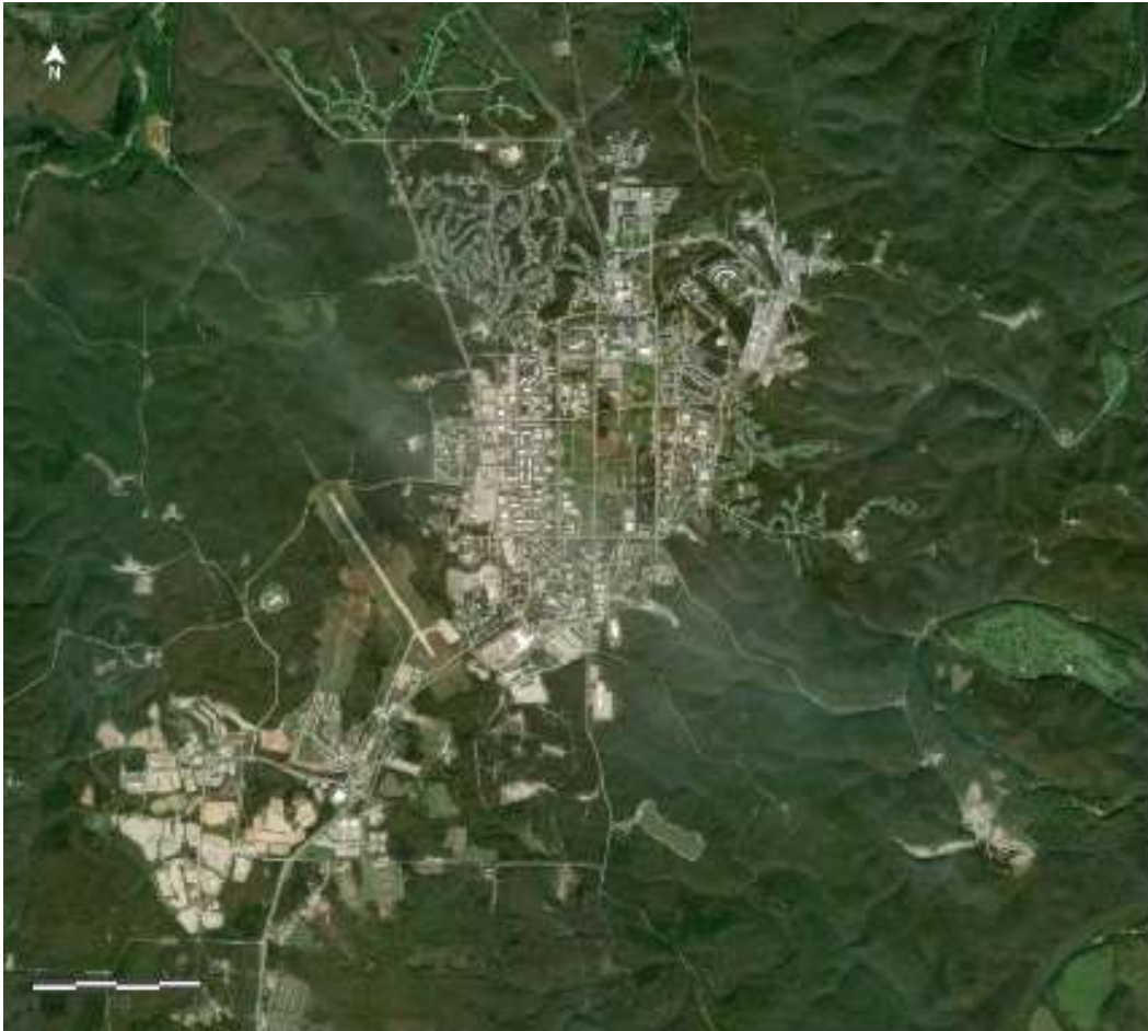
Figure 5-1. Aerial view of Fort Leonard Wood, MO (ESRI 2021).
