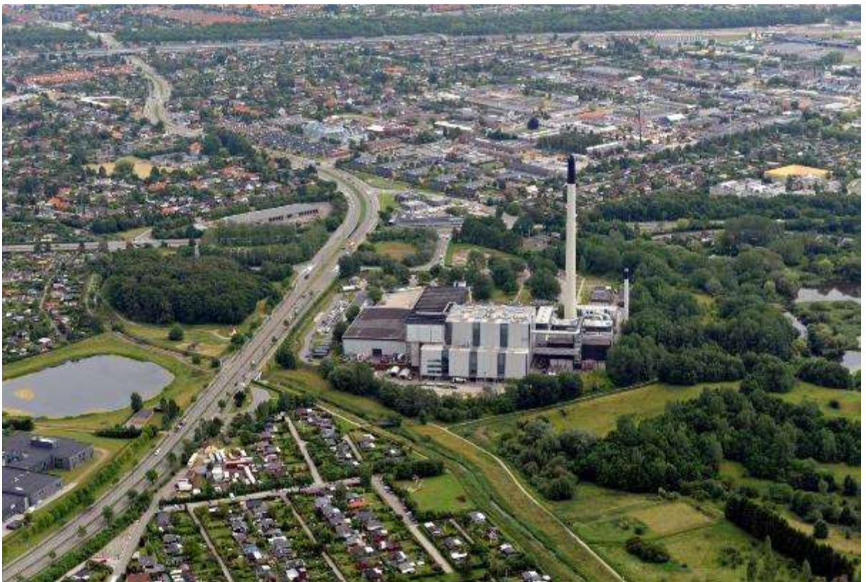
Figure 5-34. Vestforbrænding incineration plant a natural part of the urban environment.
