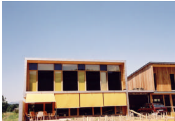
Fig. 5: 28 m 2 collector area in the façade of a wooden building, DHW and Space Heating. Wooden cover strip.
