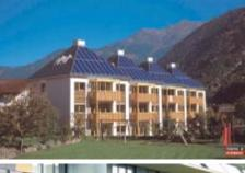
Balcony integrated solar thermal collectors
