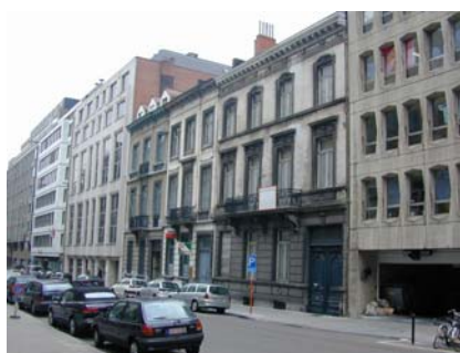
Before & after renovation
