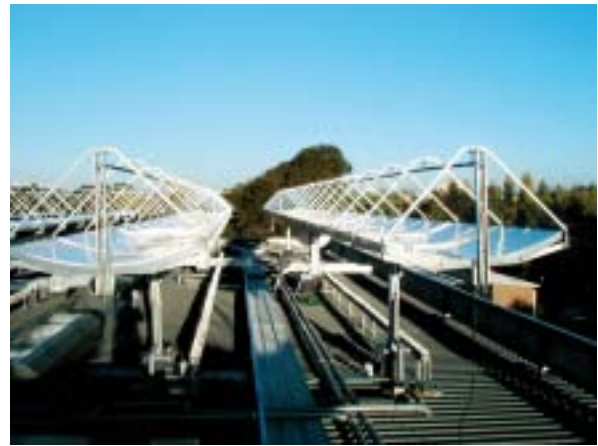
300 m 2 Bruce Hall system under construction
