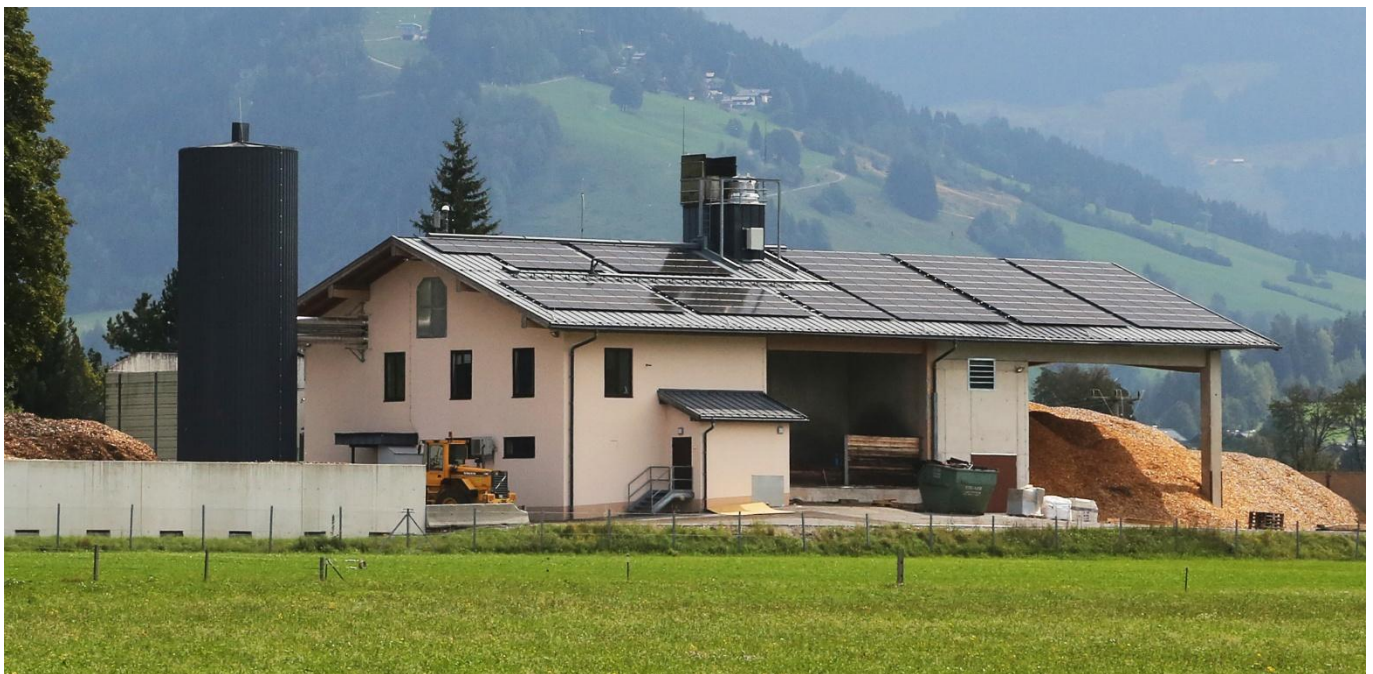
Figure 12: DH plant in Saalfelden. Source: Klimafonds / Krobath
