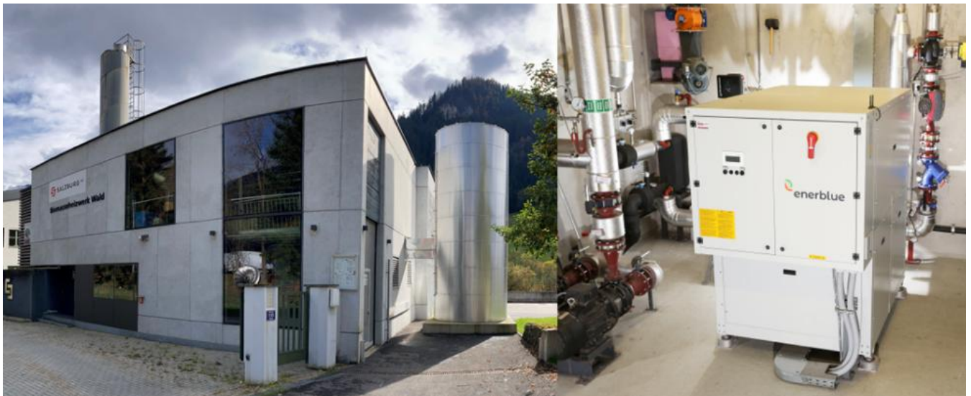
Figure 7: Left: DH plant with the 30 m 3 heat storage. Right: 250 kW th heat pump installed in the boiler house. Source: Klimafonds / Krobath
