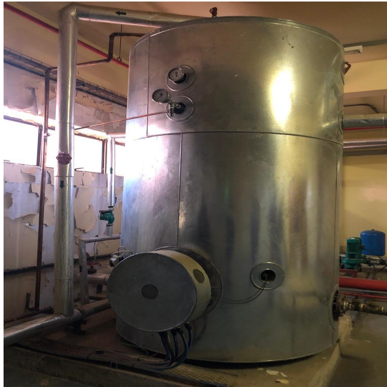
Fig 1: A storage tank boiler at the Indoor Sports Centre
