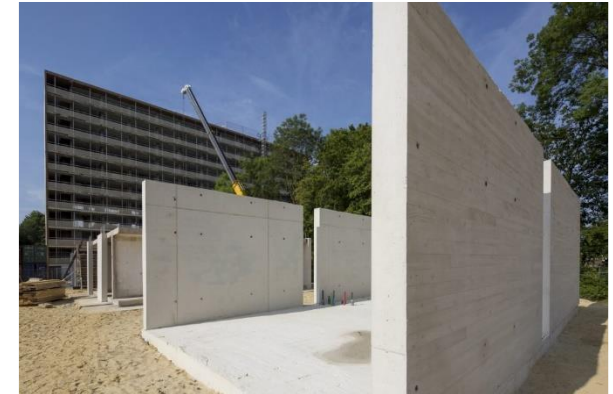
Structural elements made of circular concrete
