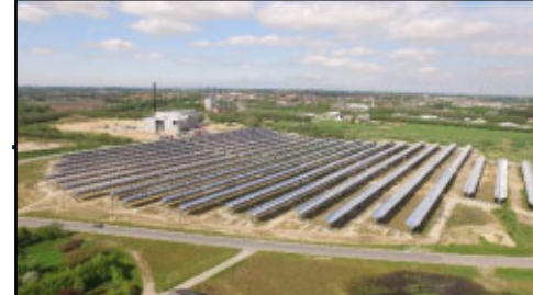
2016 CSP combined with biomass-ORC, Denmark
