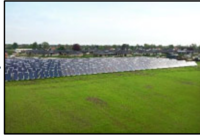
2017 Different district heating projects with flat solar panels, Denmark
