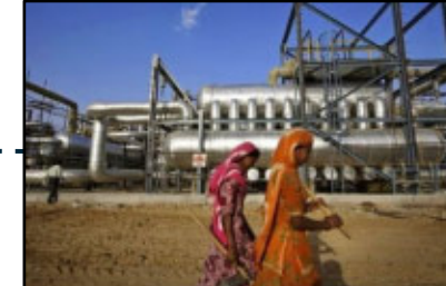
2013 50MWe and 25MWe steam generators, India
