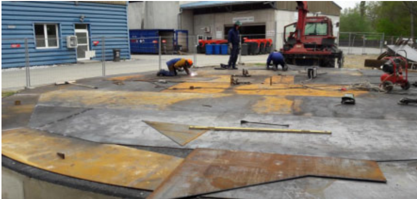
Start of tank building
