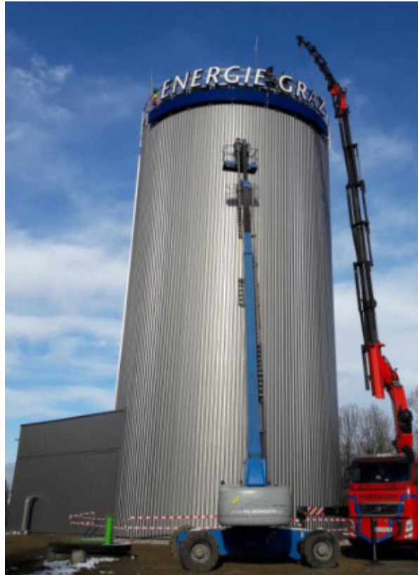
Finished storage tank with logo
