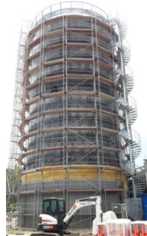
Finished tank while insulation and sheet metal cladding
