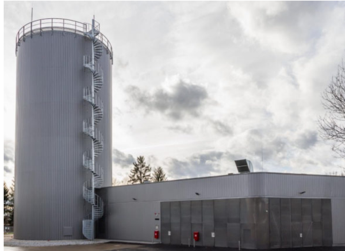
Technique center & storage tank
