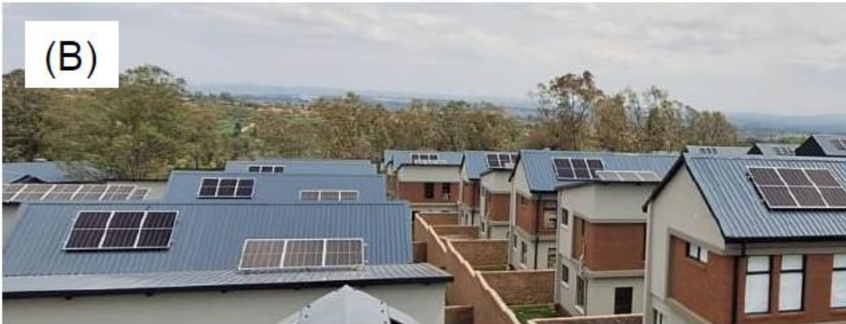
Figure 2. PV2Heat systems. (A) Market development in South Africa between 2018 and 2023 Source: Lavhe Maluleke, Stellenbosch University, South Africa; (B) Typical PV2Heat installations in South Africa, Photo: Lavhe Maluleke, Stellenbosch University, South Africa.
