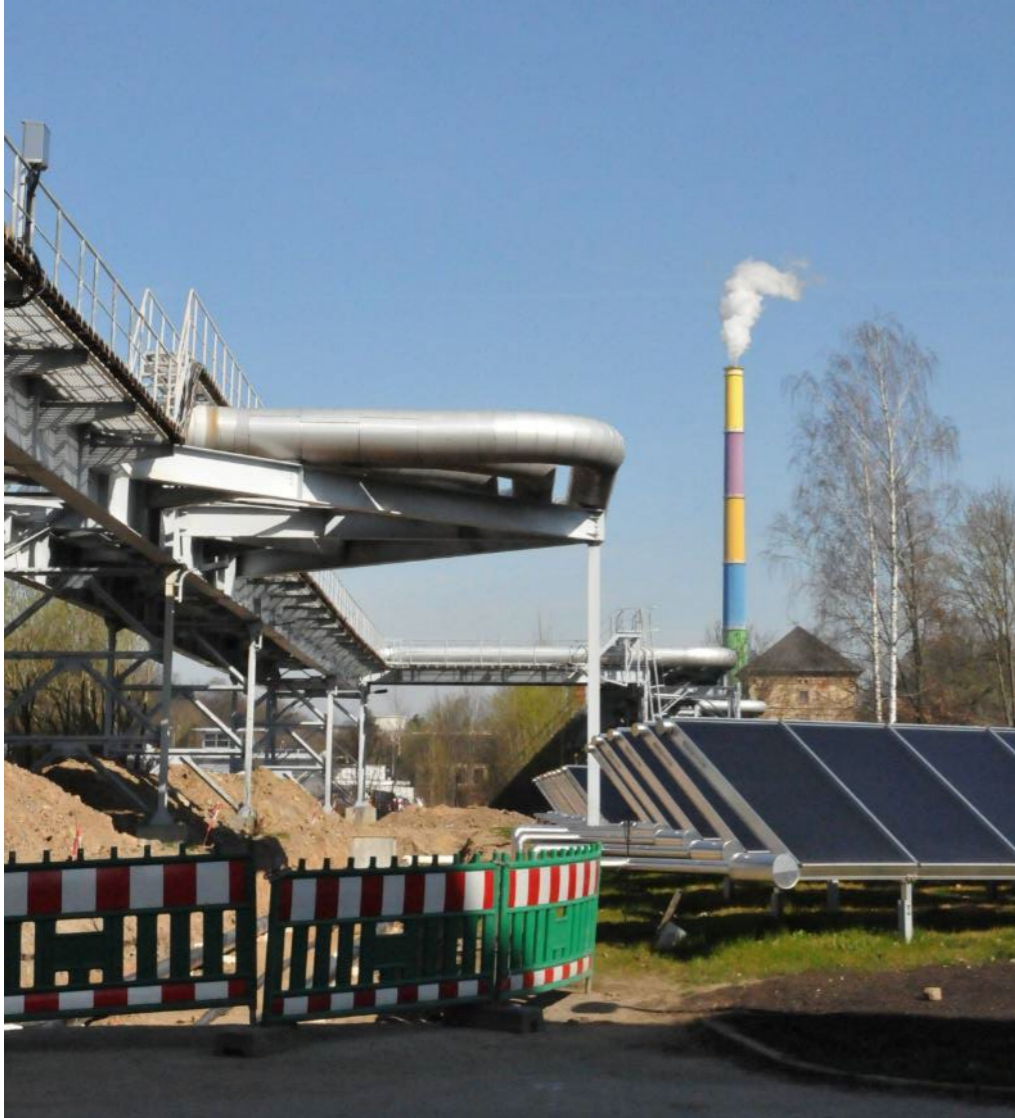
DH pipe construction in Chemnitz, source: AGFW
